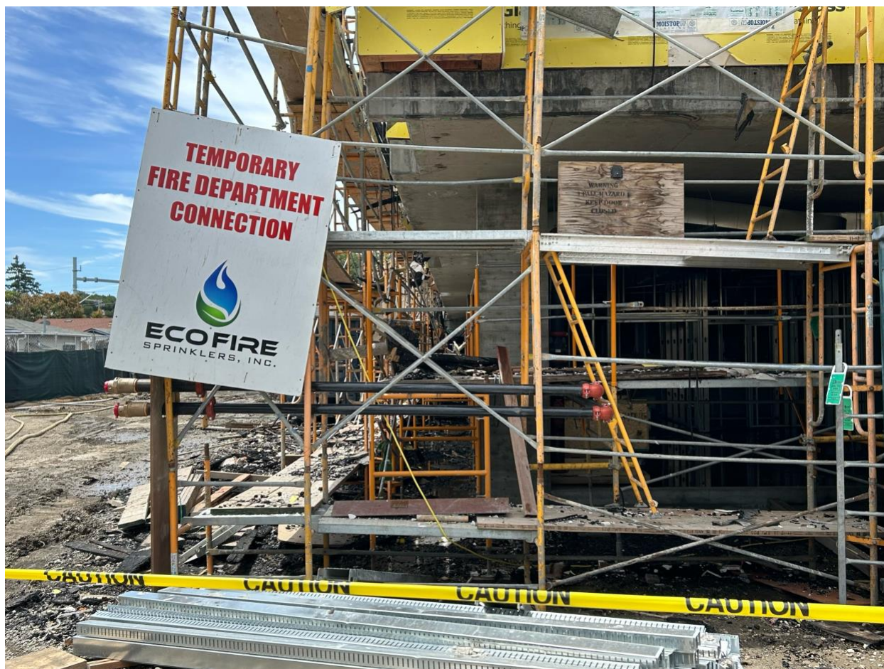
Figure 7. Temporary FDC for Building B located at the Alpha/Bravo corner.
