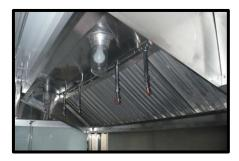
All automatic fire extinguishing systems for the kitchen hood shall comply with Underwriters Laboratories Standard 300 (UL 300). These extinguishing systems shall be serviced every 6 months. Proof of service shall be visible for fire department inspection. Vehicles with kitchen hoods must also have a class K fire extinguisher.
